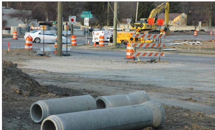
The road construction and widening project on Rochester and Wattles Roads started in February and will continue through the summer of 2010. More details about this and other road projects are on pages 10-11.
